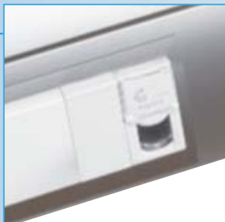
Connection of medical appliances with the Cat. 6A FTP socket.
