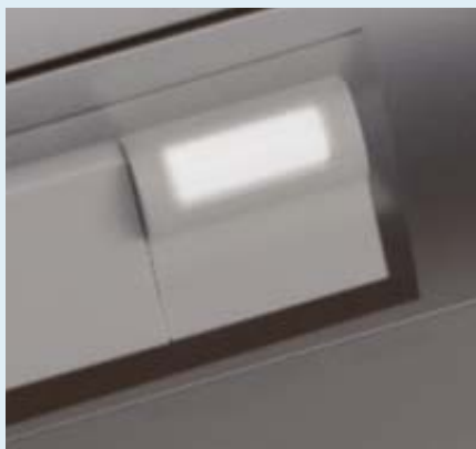
Signalling bulkhead light with low-intensity lighting integrated into the bedhead strip.
