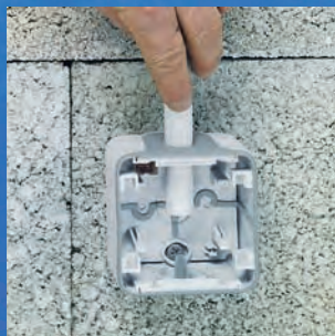
2/ Insert the tube through the end cap
