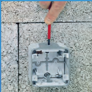
1/ Pierce the end cap using a screwdriver
