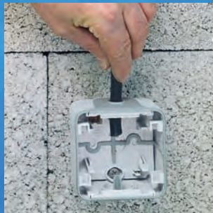
2/ Insert the cable through the end cap
